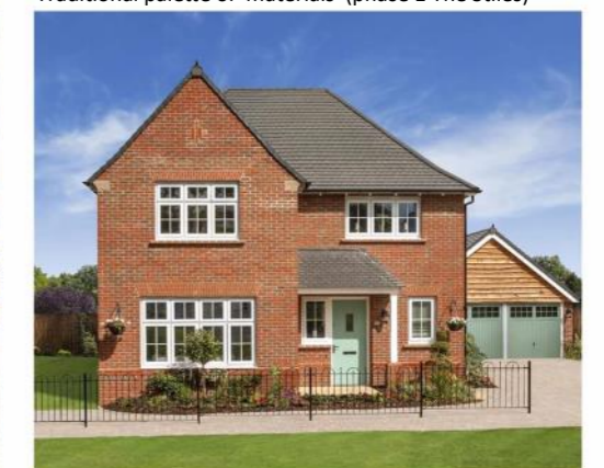
Simple but effective features and detailing
