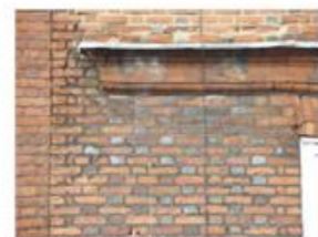
Red Brick with burnt headers: Flemish bond
